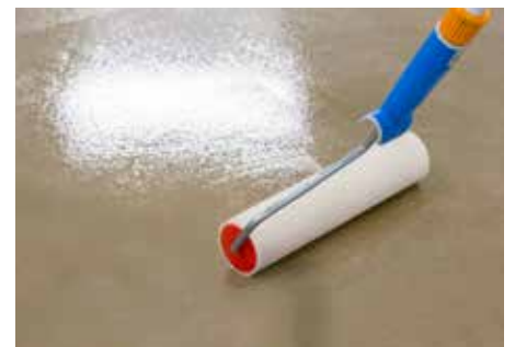
Impregnating agents based on PMCO-CT are easily applied by wiping or rolling.
