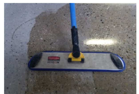
Impregnating agents based on PMCO-CT are easily applied by wiping or rolling.
